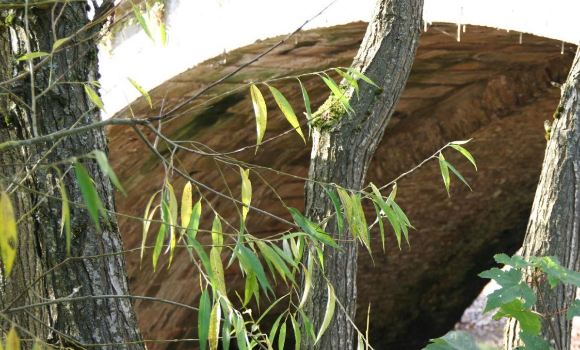
Image 6 – Grinton Bridge – n.b. narrow, rougher stonework to right
